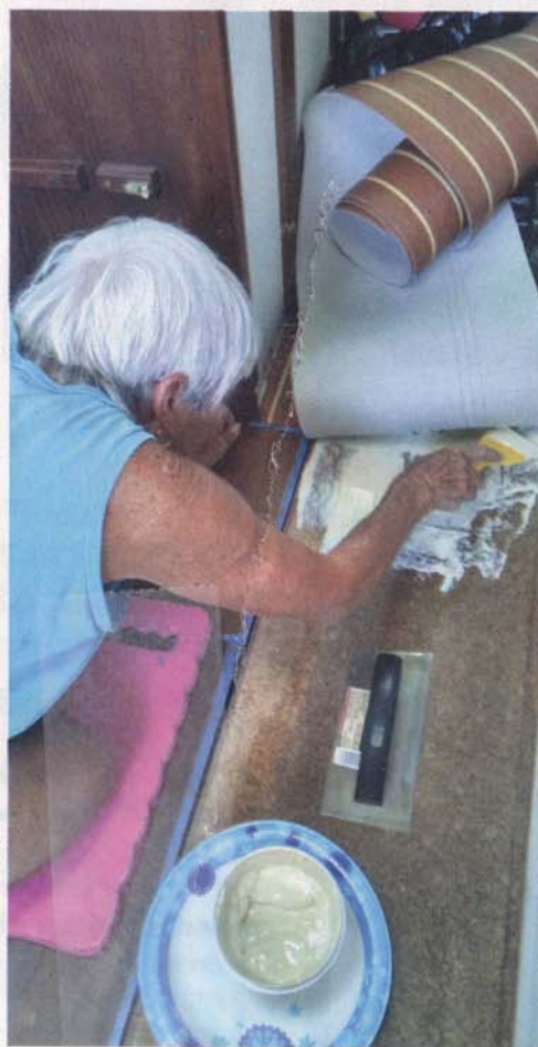
Top, the Lonseal vinyl flooring is flexible and can conform to the shape of the hull. Above, Kathy applies adhesive to the old cork sole material.
