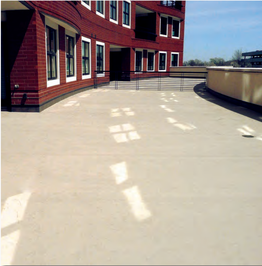
Londeck Sierra #D721 Sierra Cliff Face - Crescent Condos, St. Louis, MO
