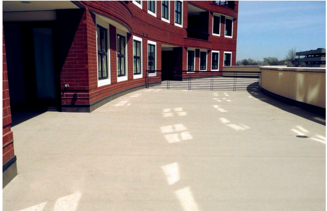
Londeck Sierra #D721 Sierra Cliff Face - Crescent Condos, St. Louis, MO
